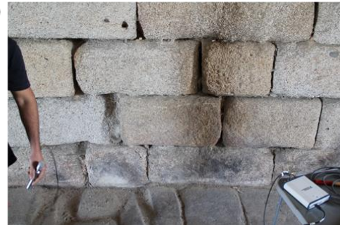
Figure 3: Current state of conservation of the Master Gate: a) main façade on which is possible to observe the strong biological colonization (orange lichens); b) detail of the current state of the barrel vault with presence of black and white crusts and; c) detail of the material losses in the lower part of the supports.
